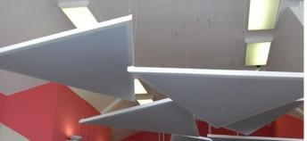
Acoustics India offers suspended roof absorbers designed to reduce reverberant noise in large open areas. Our roof absorbers are an effective and economic alternative to installing a full suspended acoustic ceiling. It is widely used in large domestic as well as industrial areas.
